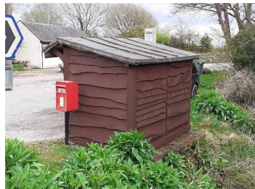
Sandyhills Bus Shelter
